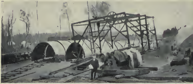
Inside forms and carrier for outside forms.
